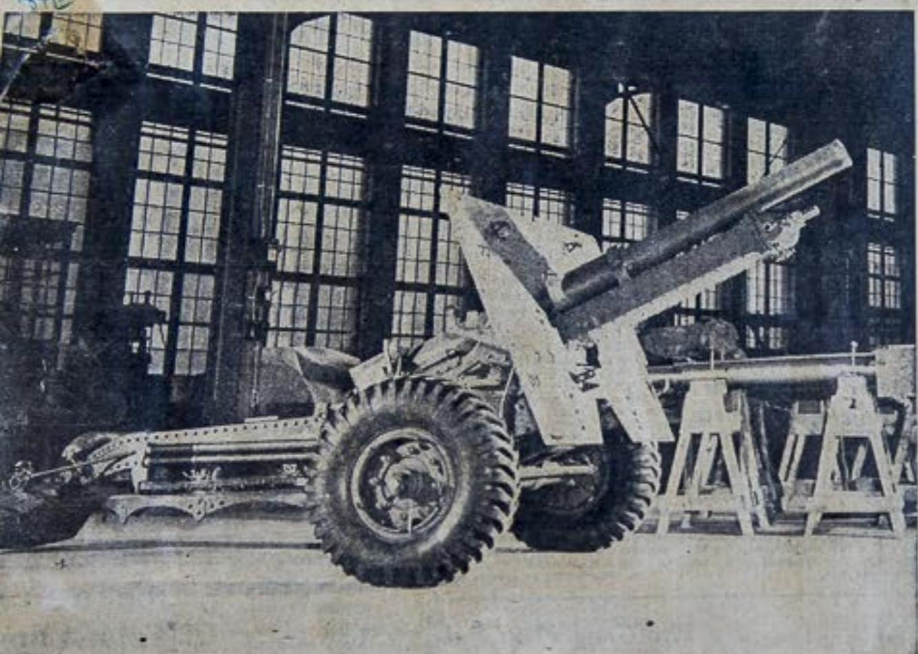
is one of the new 25-pounder guns that are being made at Sorel. The guns are being produced by Sorel Industries with the Chrysler Corporation helping by directing plant
